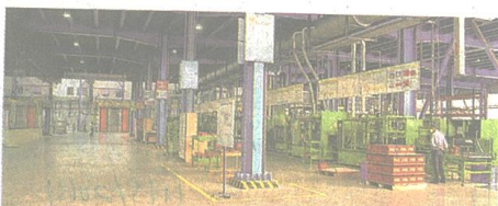
Exide's punched grid battery manufacturing unit at Haldia
