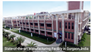
State-of-the-art Manufacturing Facility in Gurgaon, India
