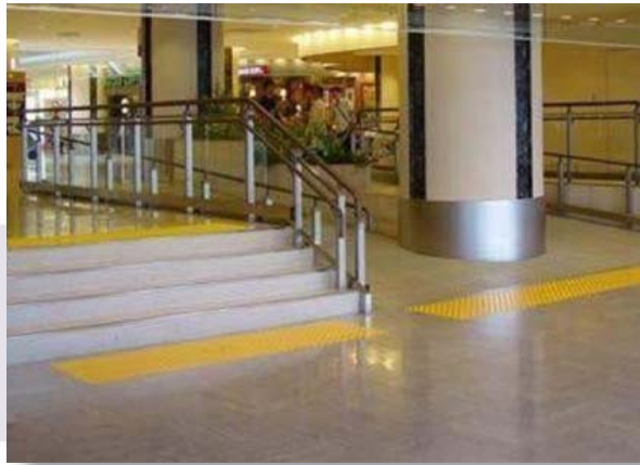
Figure 36 - Placement of Warning Blocks for Steps
