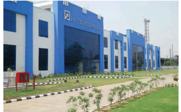
Hi-Tech Gears Green Factory Building at Bhiwadi
